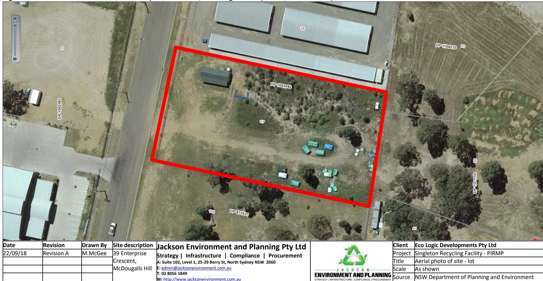
Figure 2.2. Aerial view of the lot, 39 Enterprise Crescent, McDougalls Hill (Lot 17, DP 1062083). Site boundaries are shown in red.
