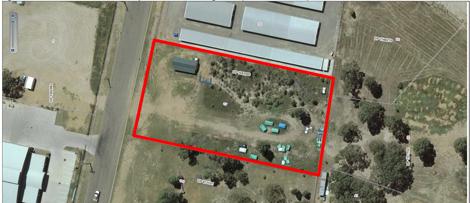
Figure 2.4. Aerial view of the lot, 39 Enterprise Crescent, McDougalls Hill (Lot 17, DP 1062083). Site boundaries are shown in red.
